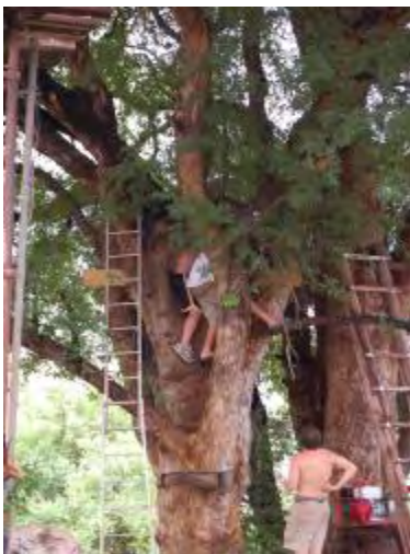
Securing the support to the tree
